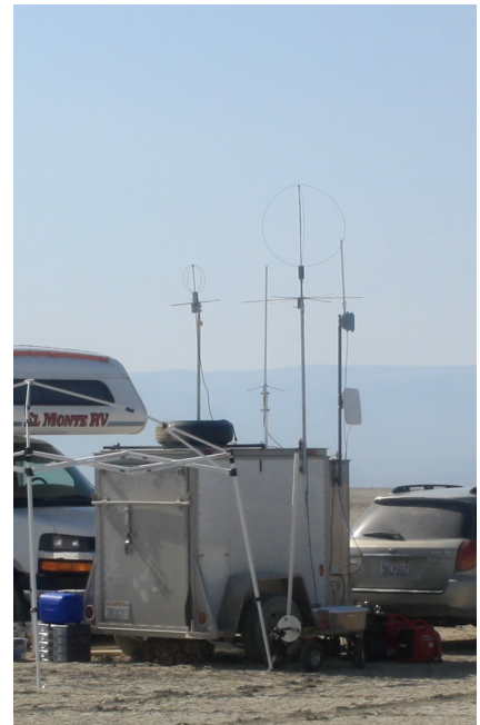
Figure 5. Base Station with APRS 70cm and 2m, 802.11a Backbone Panel and 802.11g Local Antennas.
