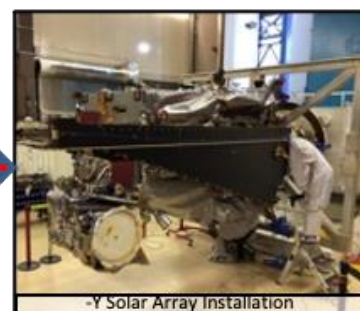
-Y Solar Array Installation
