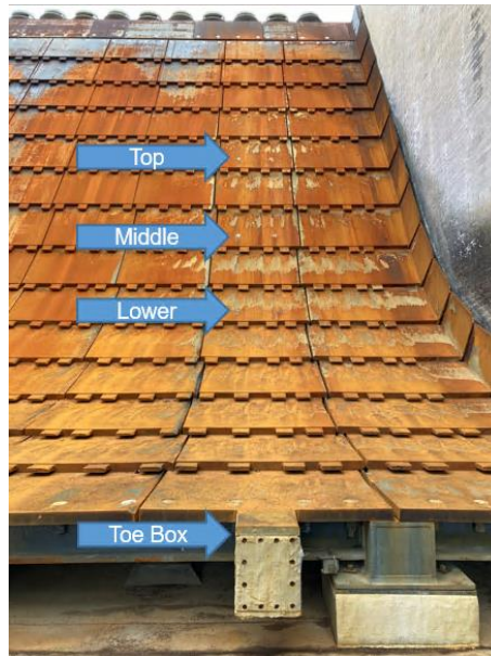
Figure 3 Artemis I Post Flight image of Ablation on Right Side of the Flame Deflector
